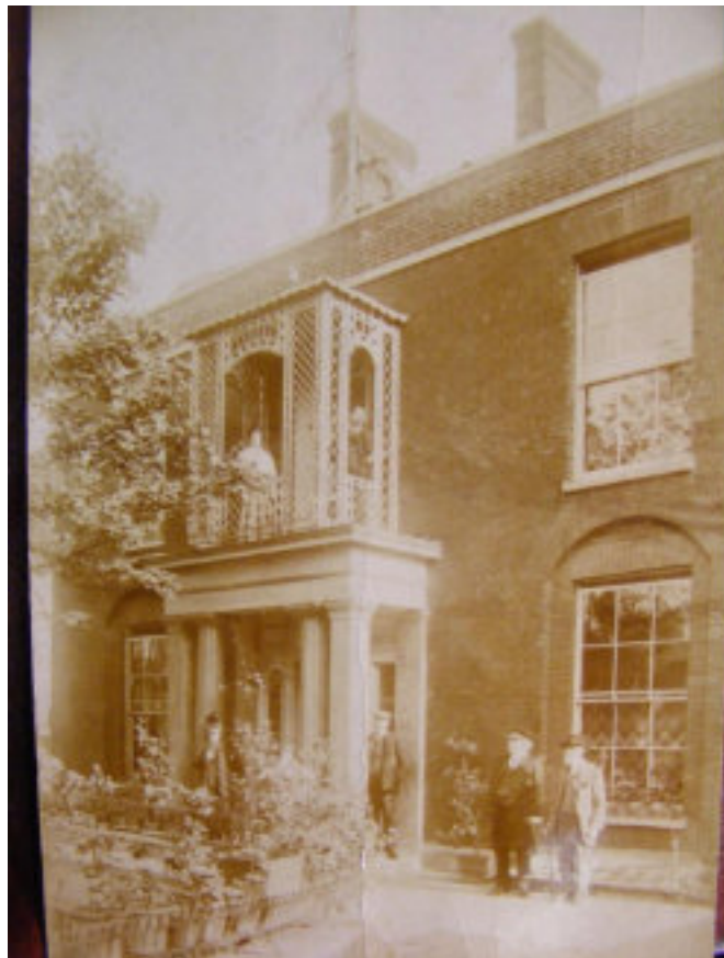
St Botolph's House, courtesy of Andrew Philips.
