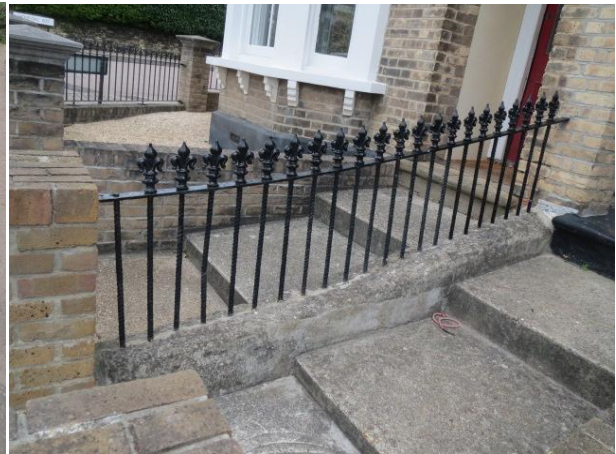
Railings at Creffield Terrace, Creffield Road.
