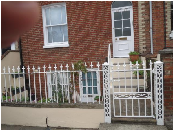
3 Roman Road railings and gate.
