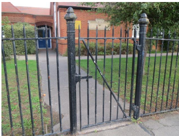
1906 Myland School gate and railings.
