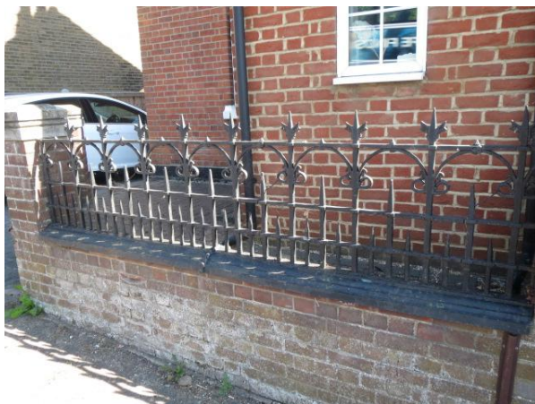
303 Harwich Road cast bases to ornate railings
