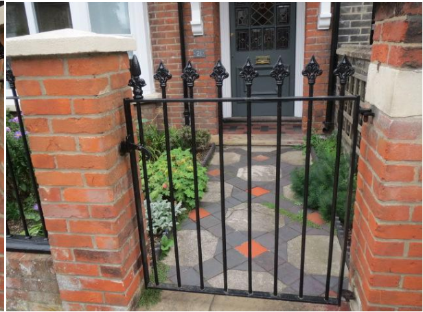
21 Roman Road ,salvaged railings with cast base re-installed. Gate made from same old railing.
