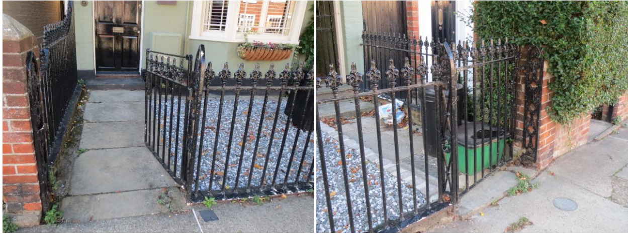
Railings and two gates with ornamental posts at 62 Castle Road.
