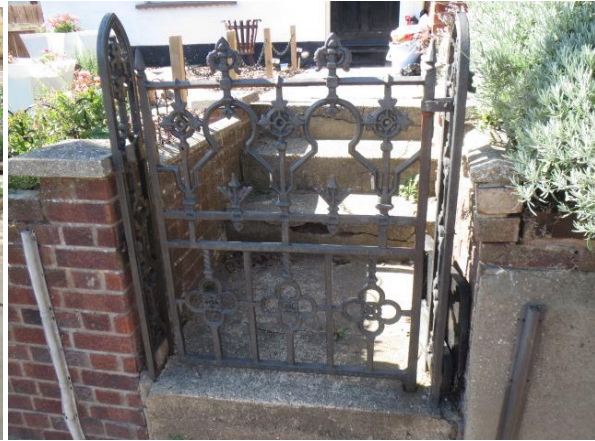
122 Harwich Road ornate gate.
