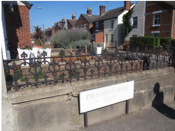
122 Harwich Road railings
