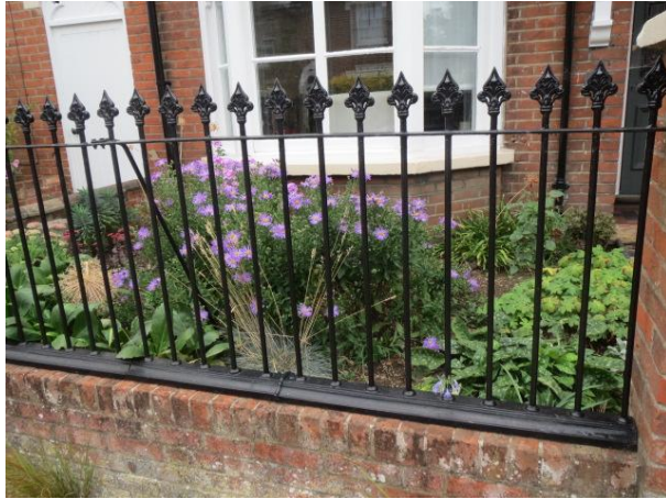
21 Roman Road ,salvaged railings with cast base re-installed. Gate made from same old railing.
