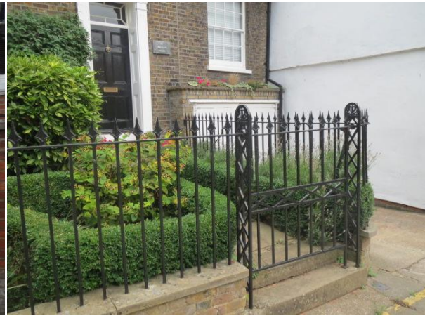
8 – 16 Abbeygate Street railings and gate.
