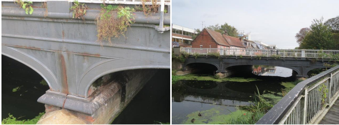
North Bridge with cast rails and pier plates and built by Coleman in 1843.
