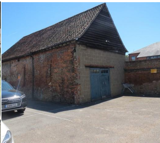
Remaining building from the Coleman foundry.
