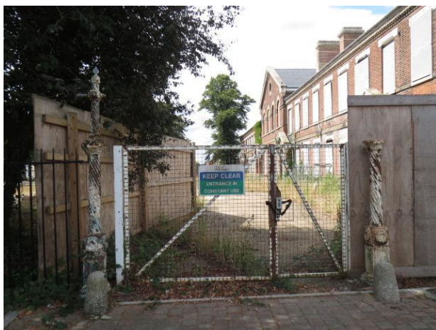
Ornate iron lamp posts at both ends of the Sergeants Mess
