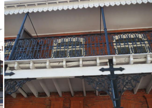
The ornate iron work veranda ,posts and brackets ,The Recreation Hotel ,Wimpole Road. Gate, posts and railings by D Rowell & Co London.
