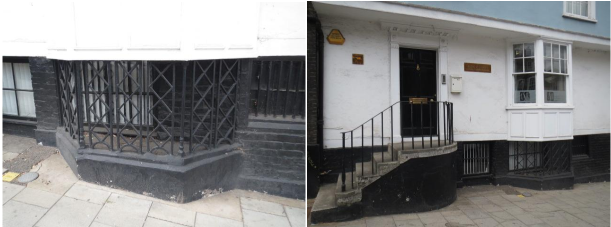
Iron Bay Supports at 57 North Hill.
