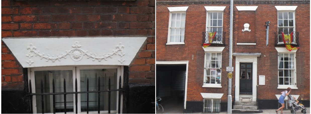
Ornate Cast Iron Lintels 5-6 North Hill, the home of Joseph Wallis ,foundry owner. Built 1809
