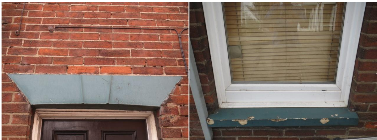
Cast Iron Lintels and Sills at 39 – 57 Barrack Street.
