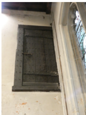
Door to the parvise room
